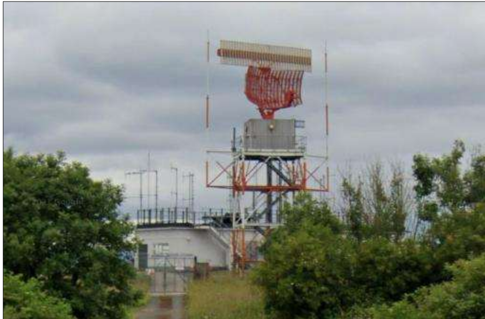
Figure 12. Dublin Airport MSSR Radar Station #1
