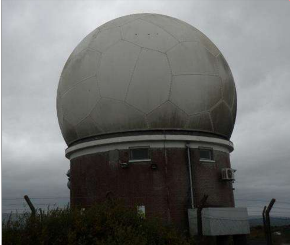
Figure 11. Woodcock Hill Radar Station
