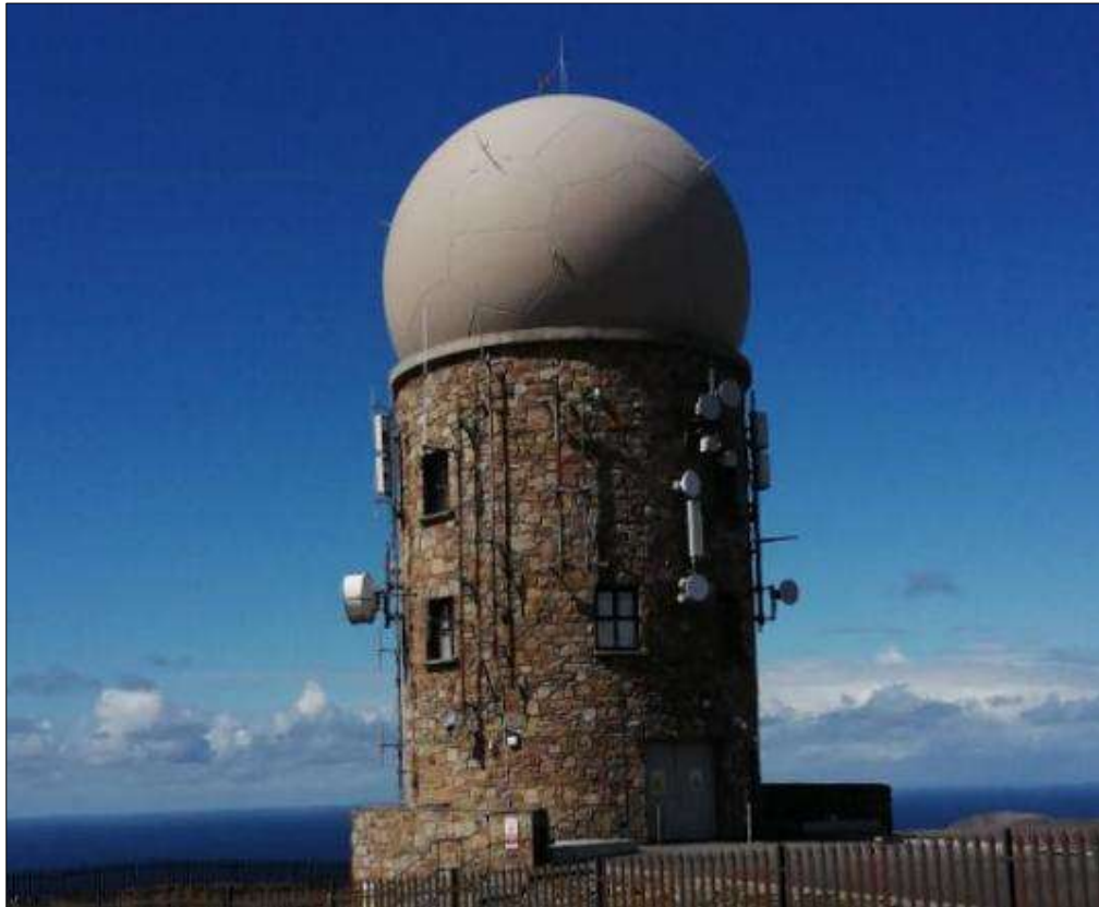
Figure 9. Dooncarton Radar Station
